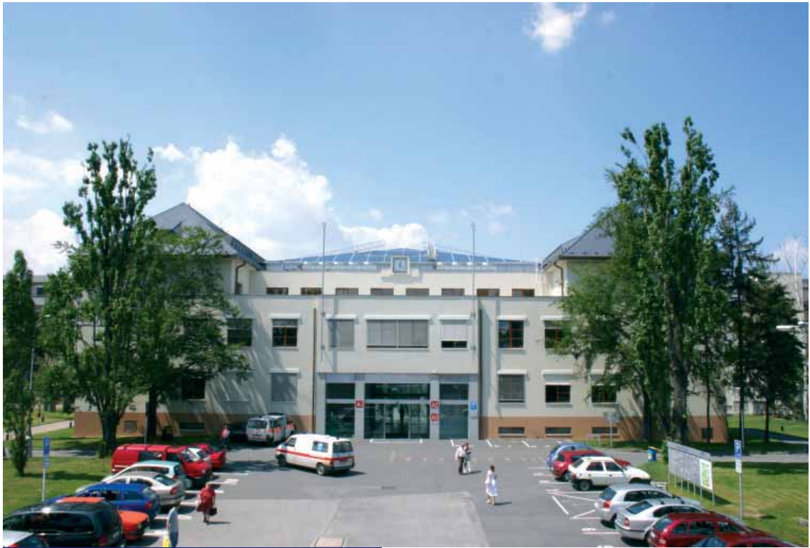
View of the newly reconstructed pavilion A
